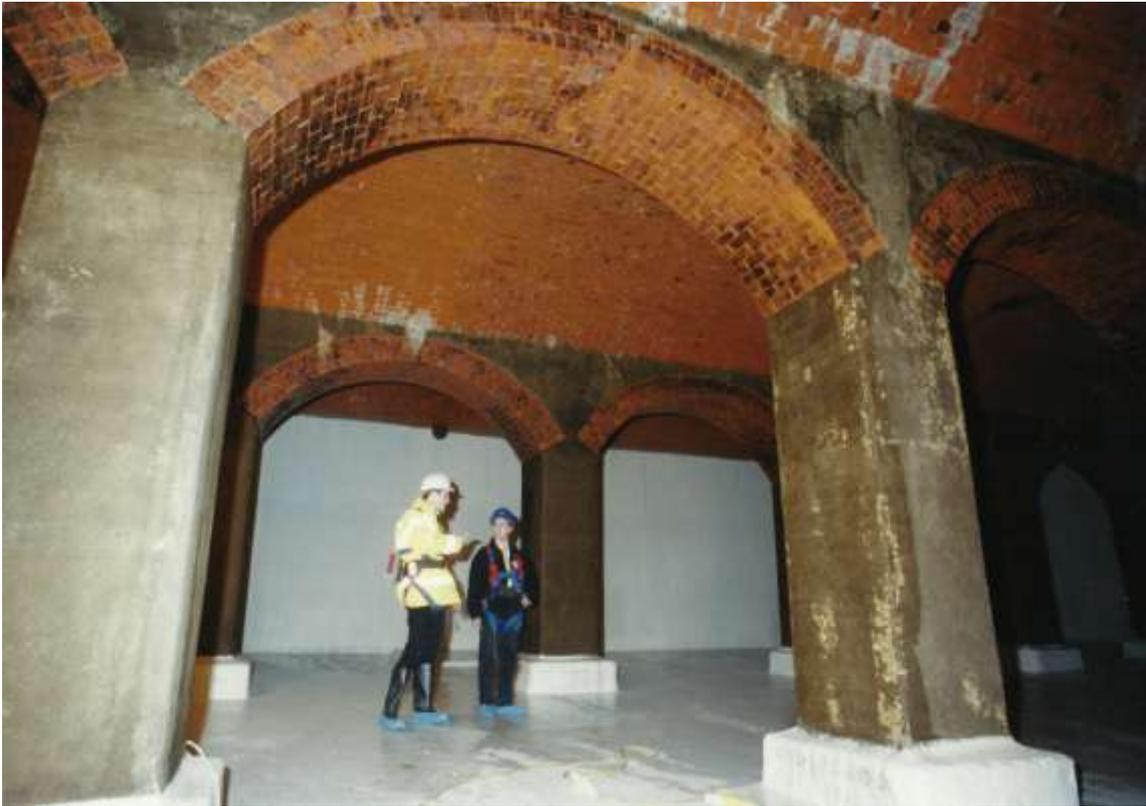
Interior of the Victoria Reservoir, Farnham, a typical covered reservoir. The photograph was taken during cleaning and renovation in 1999, 100 years after the reservoir was opened.
