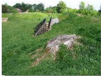
Reigate Fort: Casemate Entrance & Stumps of Felled Trees, see page 8
